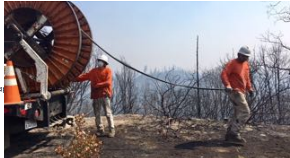
Caltrans worked with other agencies and their contractors to repair miles of damaged areas.
