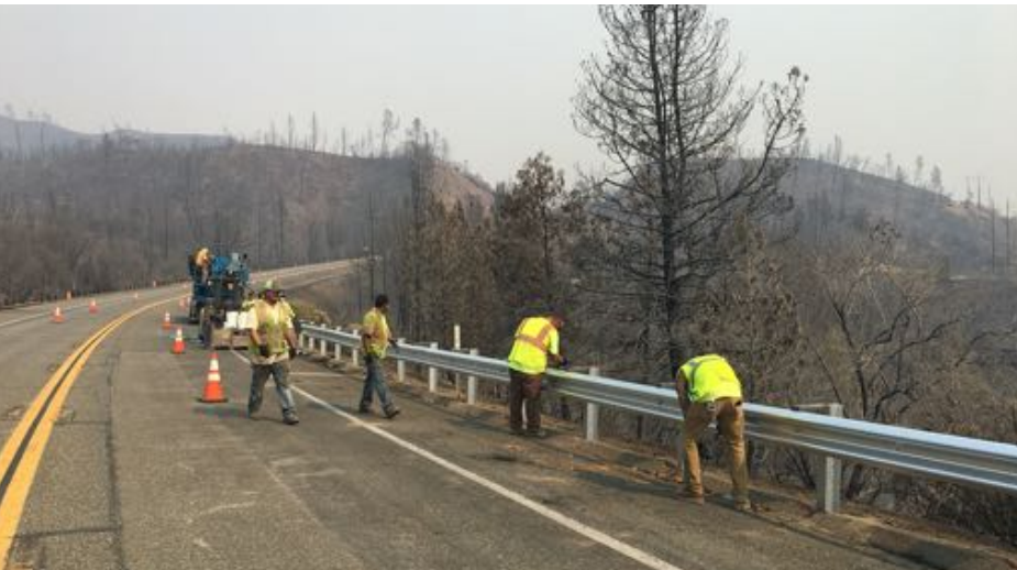
Tullis Inc. and subcontractors worked 24/7 to rapidly repair miles of burnt guardrail on State Route 299
