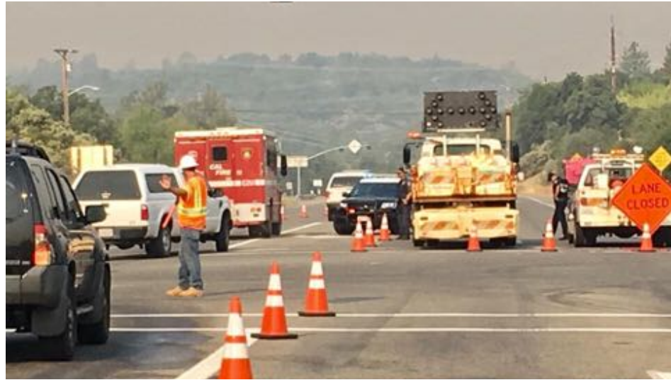
D2 Maintenance assisting with road closures in Shasta County.
